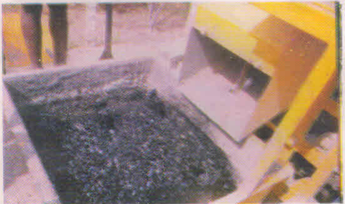
Photo – 6 Showing Polymer-Bitumen Mix.
